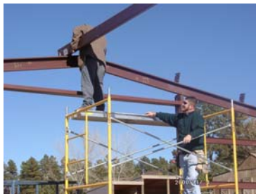
Attach the purlins to the main frames
